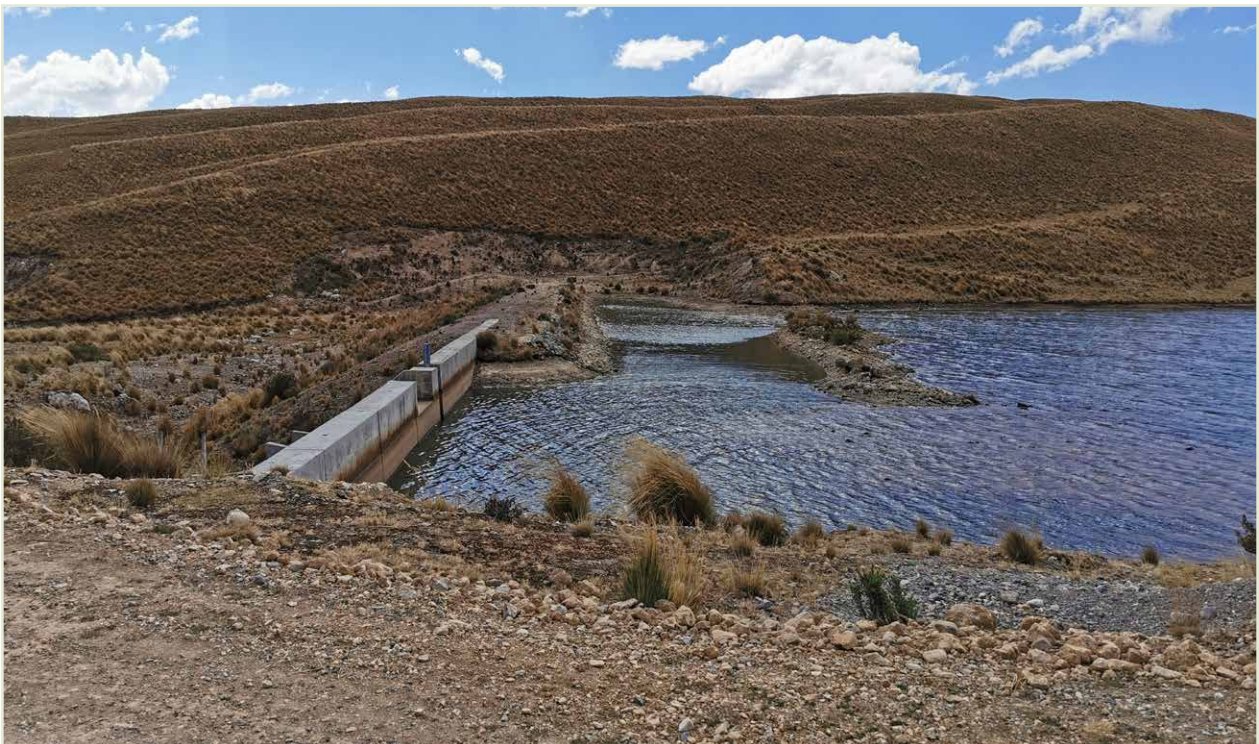
Palcash 2, a water dam in Pasco
